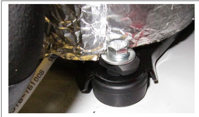
Fig. 3.3:Vibration base for compressor
