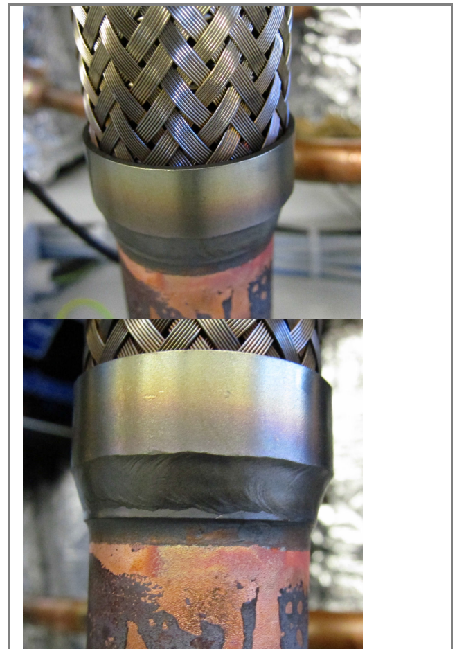
Fig. 3.5:Vibration absorber
