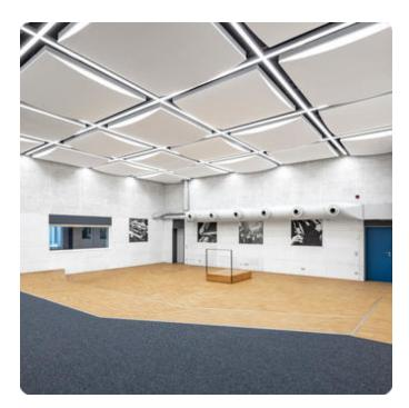
current. 1674lm. 17W. 1,8kg. Binning initial <= MacAdam 3. IP20. Protection class I. CE, UKCA marking. Prüfzeichen: ENEC. IK02. 220-240V. 50-60 Hz. RG0 (EN62471). Luminous flux reduction up to 0,4%/1.000 operating hours. Nominal failure rate: 0,2%/1.000 operating hours. L80B10 (tq 25°C) = 50.000h. 5 years warranty. Manufacturer: Lightnet GmbH, ISO 9001:2015 and 50001:2018 certified.
