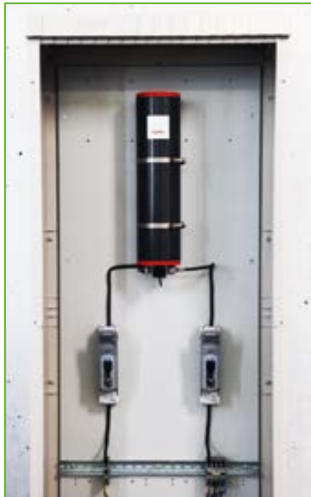
Fig. 4.4 with switch disconnecter
