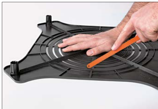
Sawing the SpotClip-Plate to size.
