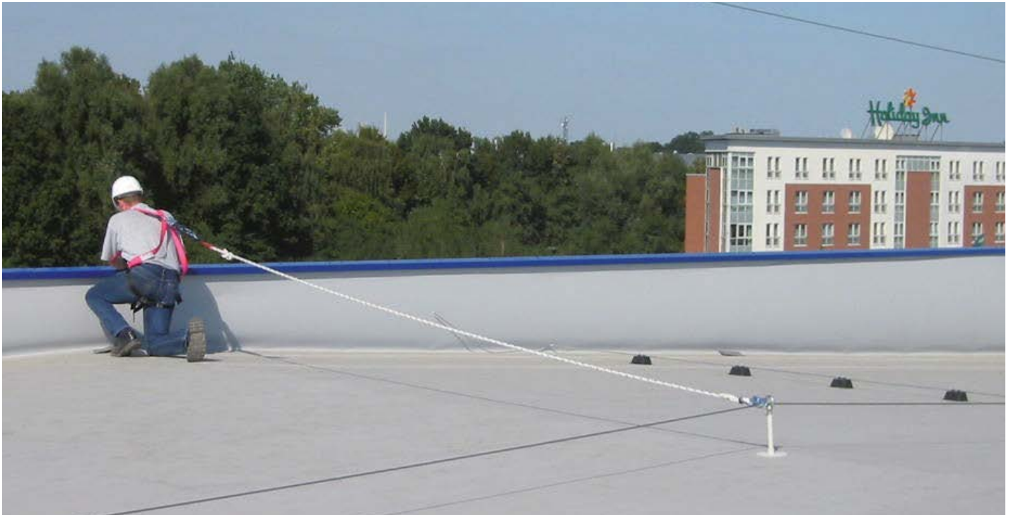
Fig. 2a Safety rope system, flat roof
