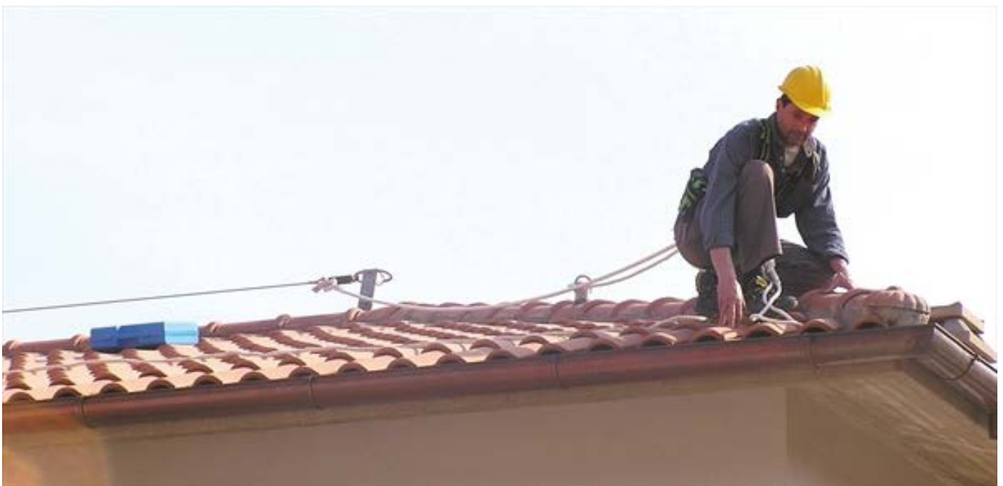
Fig. 2b Safety rope system, gable roof
